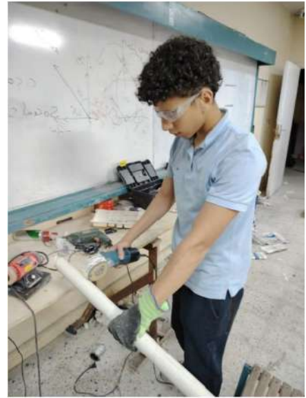
Figure 34: Safety measures taken while working
